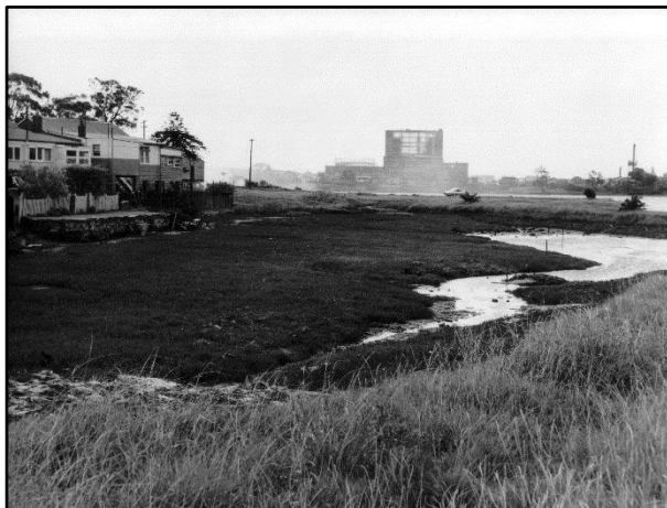
Figure 15. Bushells Factory, c. 1966, without chimney. 33
