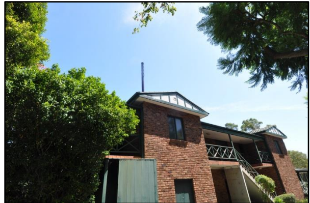
Figure 34. Eastern façade of administration building with half-timbered gables shown.
