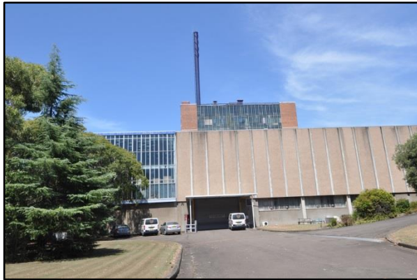
Figure 39. Detail of northern façade of factory with precast concrete panels.
