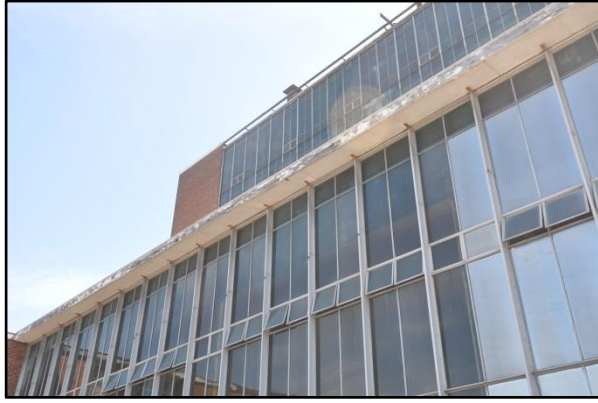
Figure 49. View of clerestory aluminium framed glazing as viewed from the second-floor roof space.
