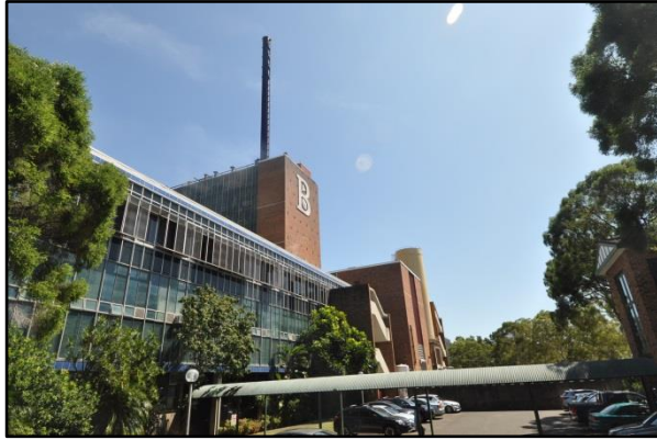
Figure 31. View of the covered walkway joining the eastern façade of the factory to the administration building.
