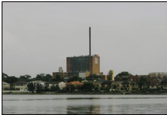
Figure 27. View of subject site from Hen and Chicken Bay, c. 2007. 62
