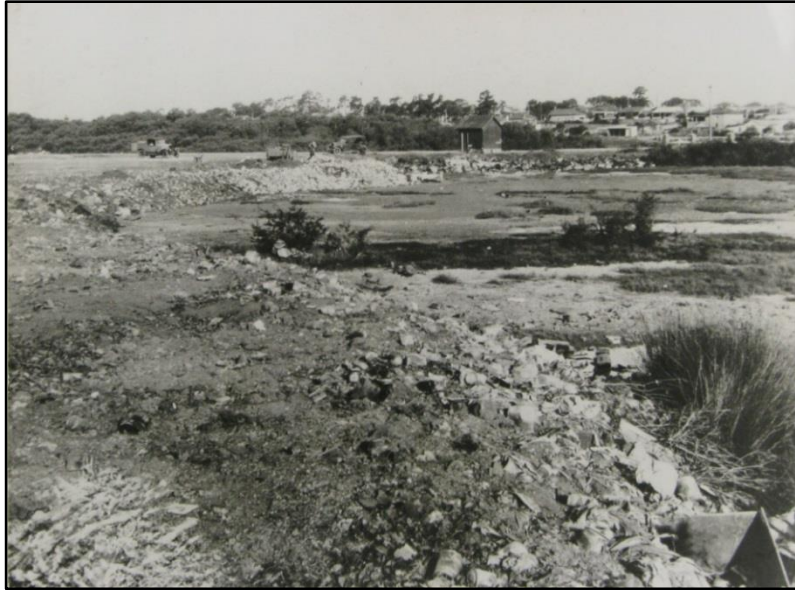
Figure 11. Reclamation works at Exile Bay, c.1930. 27
