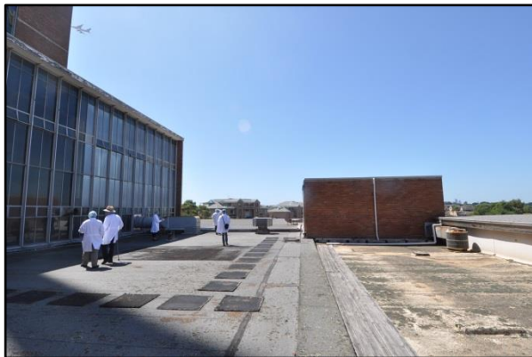
Figure 45. Roof space located on second floor.
