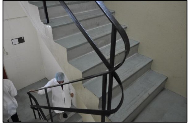
Figure 50. Curved steel handrails located in stairwell located between floor five and floor three. Despite not achieving BCA Compliance, the existing handrails should be retained and reused on site.
